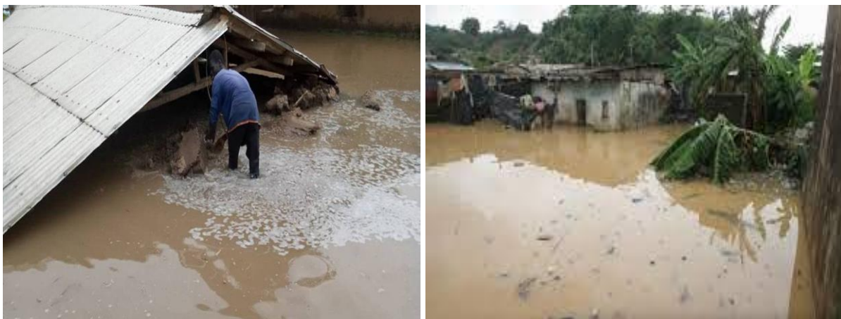
Figure 119: destruction of houses due to heavy rains on 11 and 12 November 2020 in Béwondo
