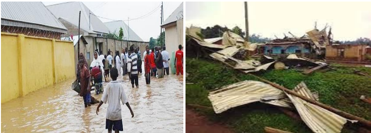
Figure 120: illustration of cases of flooding in the New-Bell district of Ebolowa and the destruction of school infrastructure in Obala following heavy rains accompanied by violent winds
