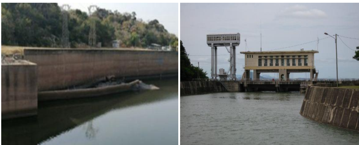
Figure 102: Drop in the water level of the Benue River affecting the production of the Lagdo hydroelectric power station.
