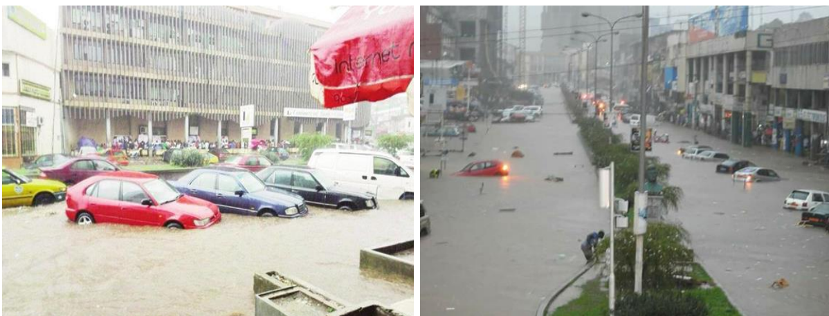
Figure 121: Significant material damage recorded in Kennedy Avenue on September 02 2020 due to flooding caused by heavy rains.
